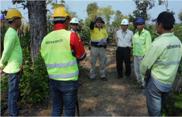
Safety brief by Ian Mulroy to Milsearch and NTPC Personnel prior to demolitions.
