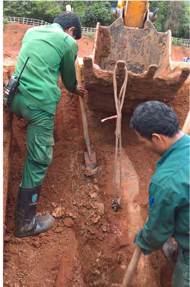
Excavation of a M117 750lb airdropped bomb found by MAG at the construction site for a market in Najat village Bualapha district Khammouane.
